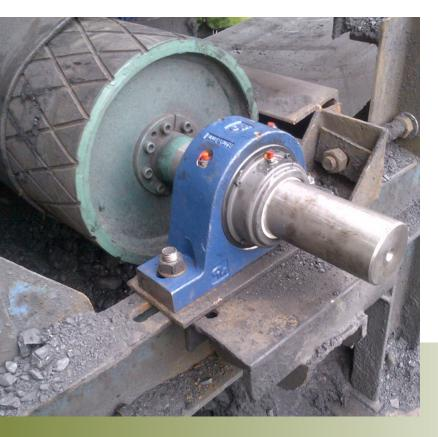
After installing two Timken spherical roller bearing solid-block housed units at the tail pulley positions, New Clydesdale decided to install more units at several locations in its conveyor system.
